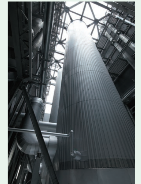
Cold water vertical thermal storage tank at Tokyo Data Center I
